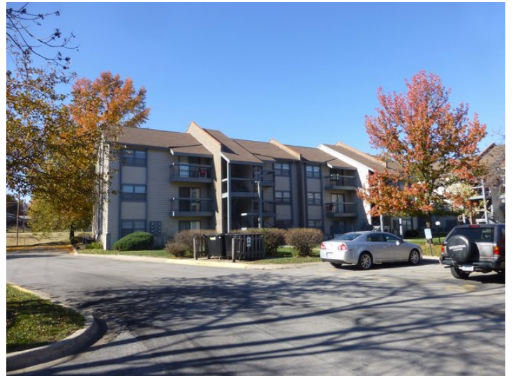
TYPICAL EXTERIOR VIEW.
