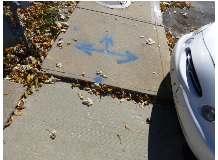
CORRECT TRIP HAZARD.
