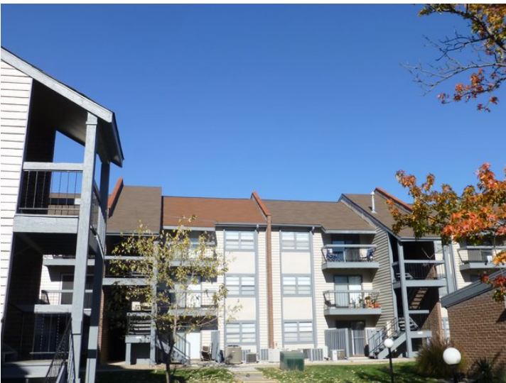
TYPICAL EXTERIOR VIEW.
