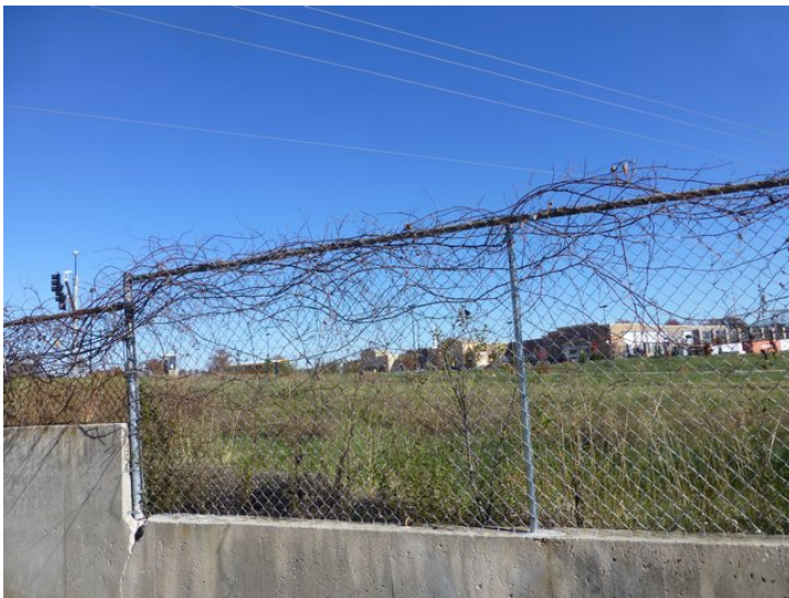
ADJOINING VIEW EAST.
