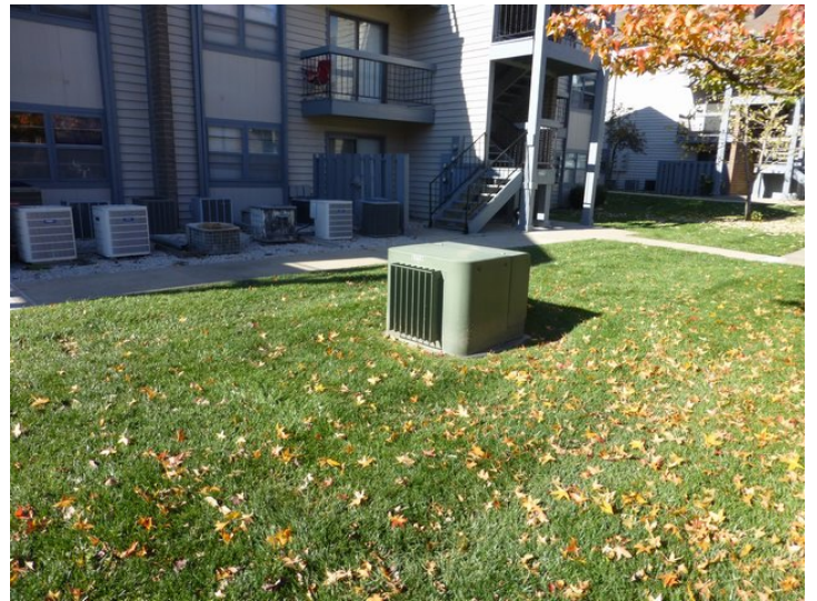
PAD-MOUNTED TRANSFORMER.
