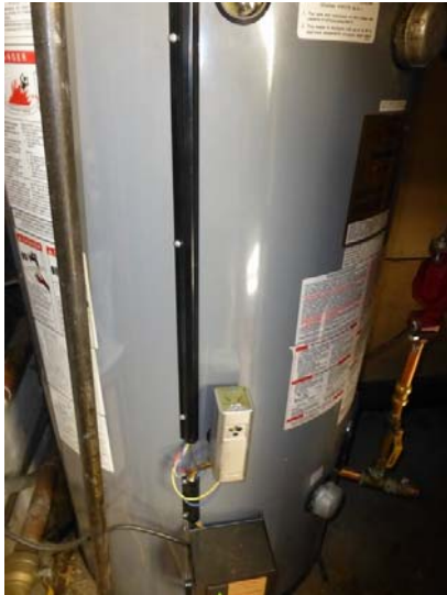
CENTRAL DOMESTIC WATER HEATER.
