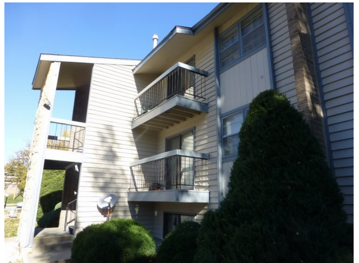
TYPICAL EXTERIOR VIEW.
