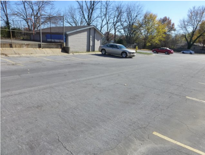
SEAL COAT AND RESTRIPE PARKING LOT.
