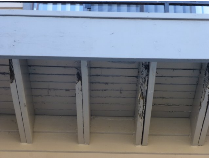
RECONDITION BALCONY SUPPORTS.
