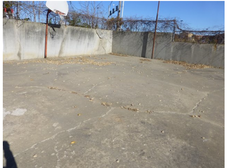
REPAIR BASKETBALL COURT.
