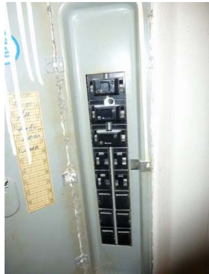
CIRCUIT BREAKER PANEL.
