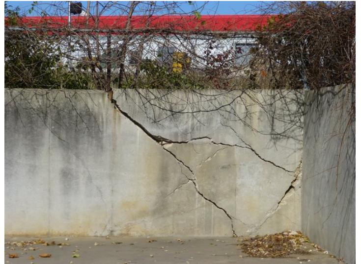
REPAIR RETAINING WALL NEAR BASKETBALL COURT.
