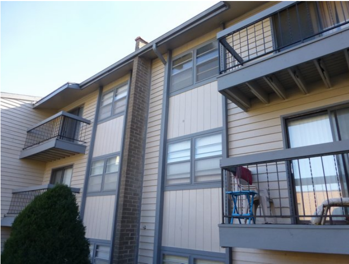
TYPICAL EXTERIOR VIEW.
