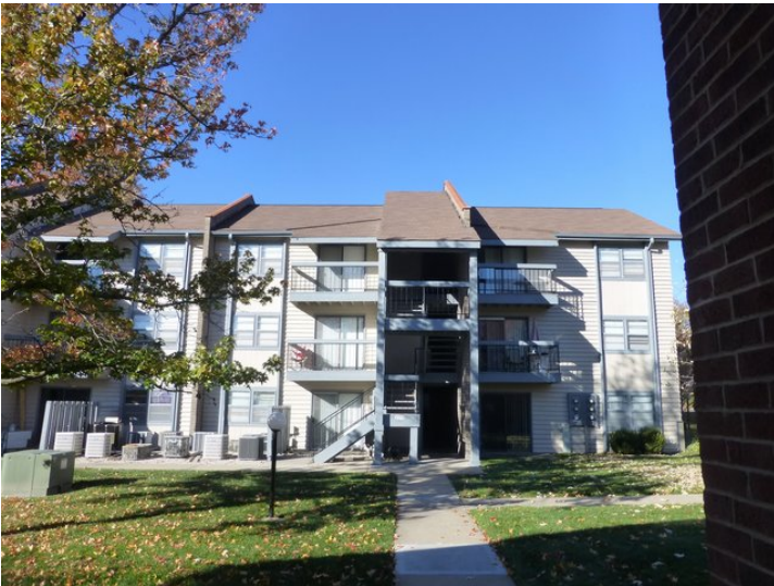
TYPICAL EXTERIOR VIEW.
