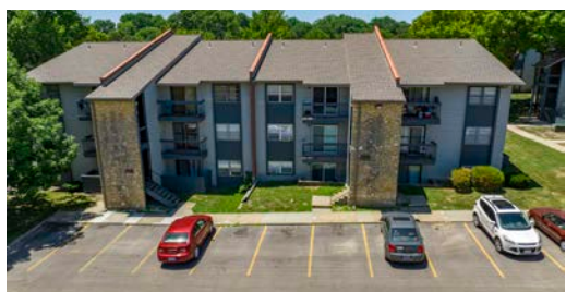
RAYTOWN VILLAGE 7705 Raytown Rd, Raytown, MO
