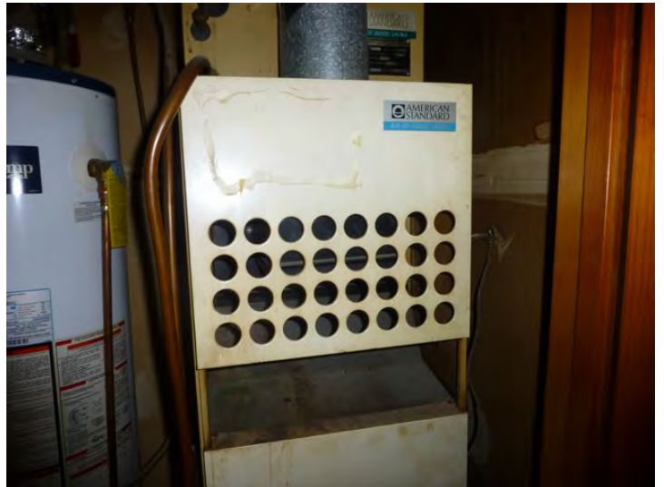
FURNACE AT UNIT.
