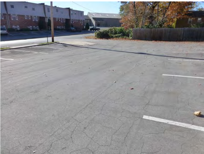
SLURRY COAT AND RESTRIPE PARKING LOT.
