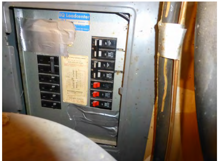
CIRCUIT BREAKER PANEL.
