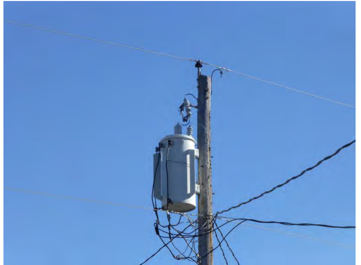
POLE-MOUNTED TRANSFORMER.
