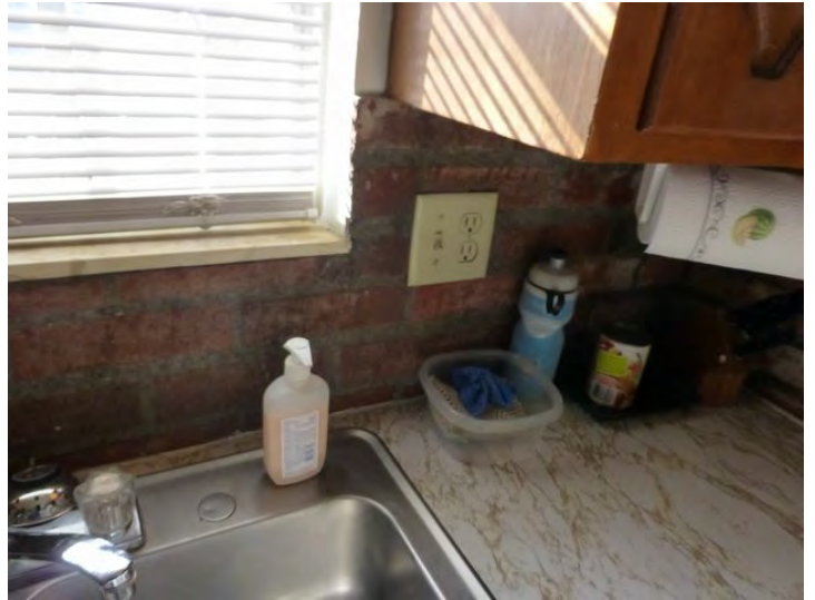
INSTALL GFCI OUTLETS.
