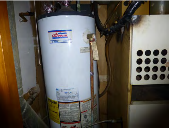
DOMESTIC WATER HEATER.
