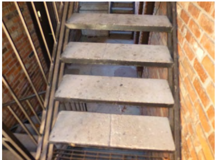
REPAIR DAMAGED TREADS AT BUILDING 7230.
