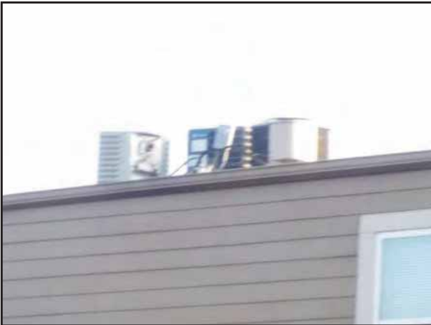
Roof mounted AC condensers were observed at the Property.
