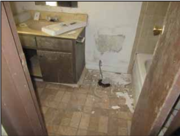
Damaged ACM and LBP materials were observed at the Property during the PCA inspection.
