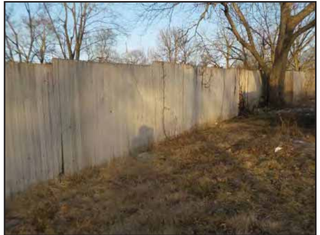
Wood fencing was observed on portions of the north and west perimeters of the Property.
