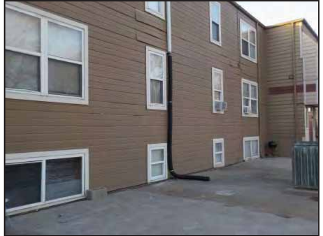
Storm water is drained from building roofs by gutters and downspouts.
