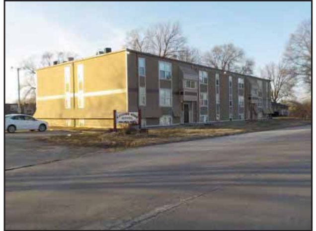
The flat roofs were reported to contain TPO and modified bitumen.
