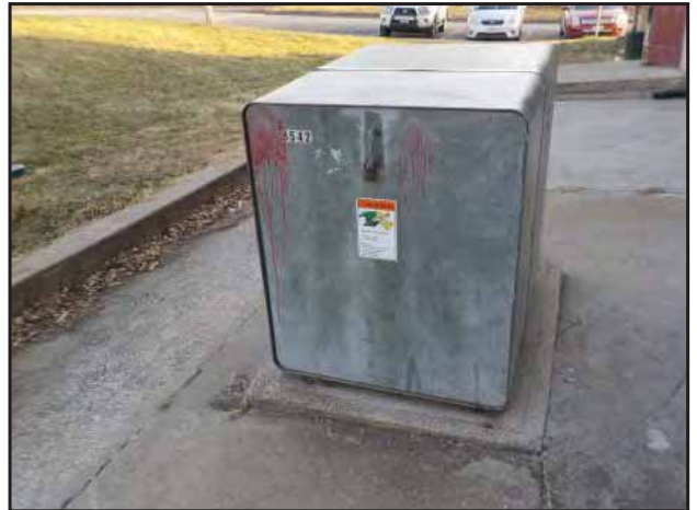
Pad mounted transformers were observed at the Property.
