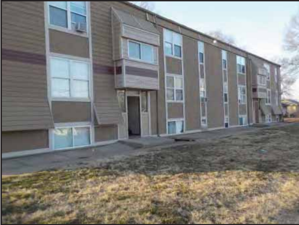
Exterior finishes consist of T1-11, composition board, and cementitious siding.
