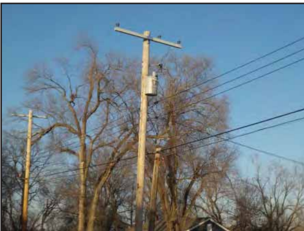
Pole mounted transformers were observed adjacent to the Property.
