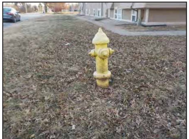
Fire hydrants were observed on the Property.
