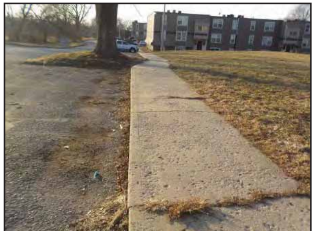
Concrete pedestrian walkways were observed throughout the Property.
