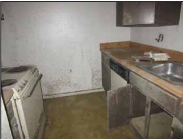
Mold was observed at the Property during the PCA inspection.
